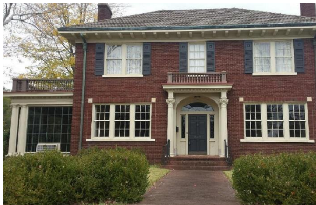
Tile roof – copper gutters – detailed millwork
